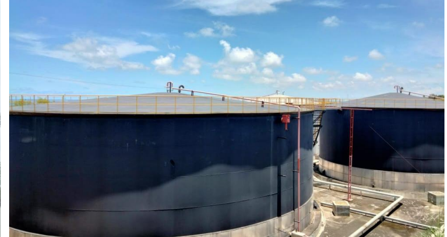
VTB and HVGO Tank Storage at LSB Port
